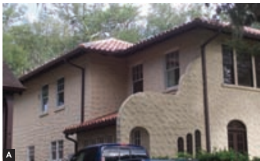
Replacement windows on side of residence.
