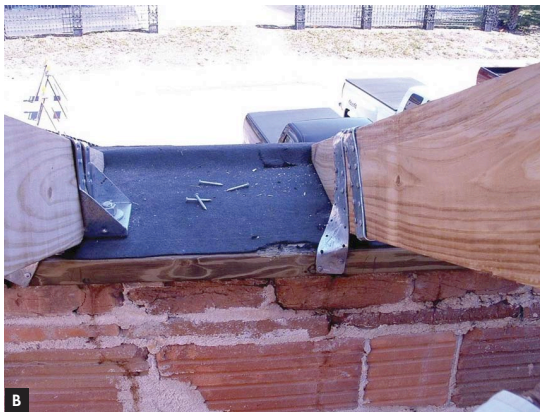
A) Front Elevation of Ringling Ca d'Zan Gatehouse; B) Rafter tie down straps/anchors in masonry wall; C) Rafter tie down straps/anchors. 1926 Ringling Estate, Ca d'Zan, Sarasota
