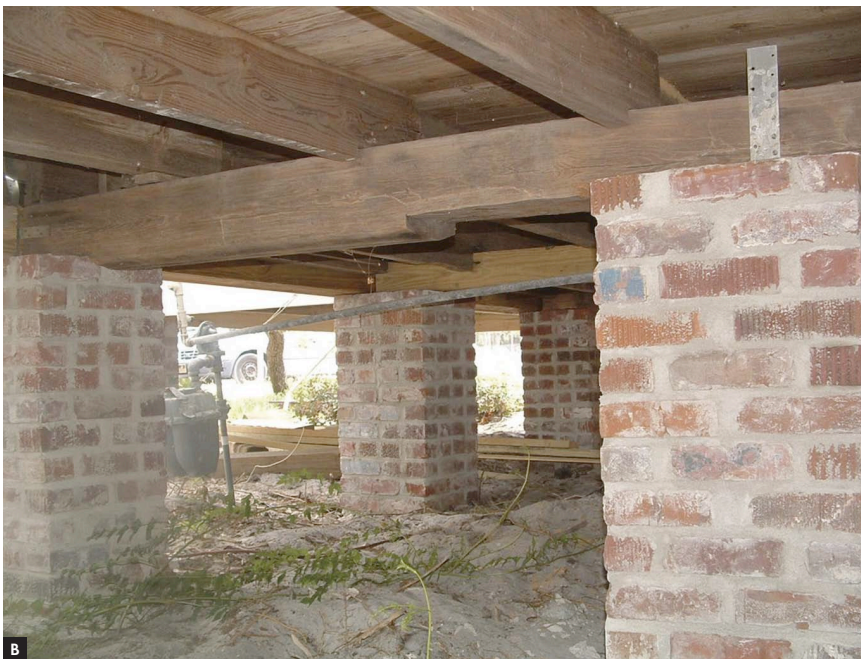
A) 1937 Maddox House in Port St. Joe; B) Sill Beam Tie Downs Trap to New Masonry Piers
