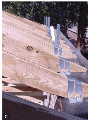
A) Front Elevation of Ringling Ca d'Zan Gatehouse; B) Rafter tie down straps/anchors in masonry wall; C) Rafter tie down straps/anchors. 1926 Ringling Estate, Ca d'Zan, Sarasota
